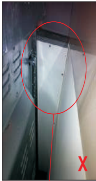
Left Side of oven, chain not attached
